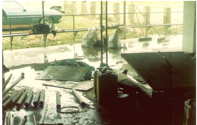
Flood debris left in clubhouse
